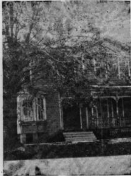
The present home of Mrs. Morgan Treat, the older portion of which was the earliest postoffice building here.
