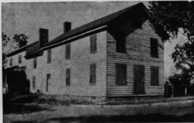
West Point's first store, built by Mr. William Mitchell. It stands at the corner of Third and D streets.
